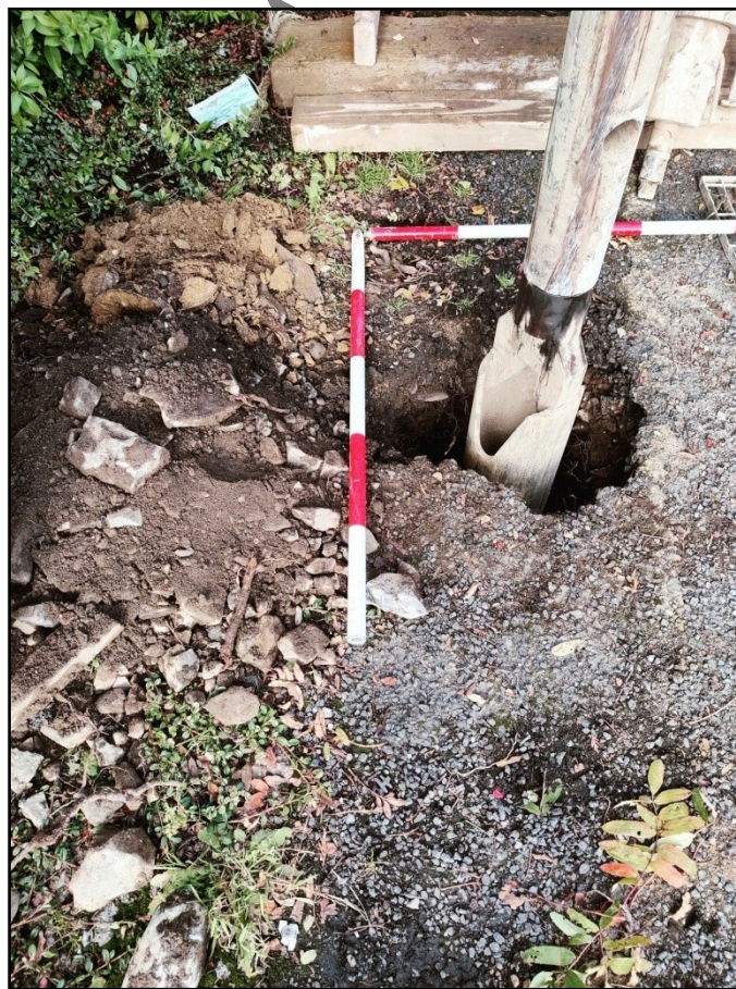
Plate 18 Cable percussion R9-CP13
