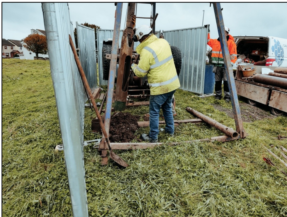
Plate 8 Cable percussion R9-CP04
